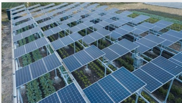
Figure 2: : Mounted solar panels shade crops growing underneath them
